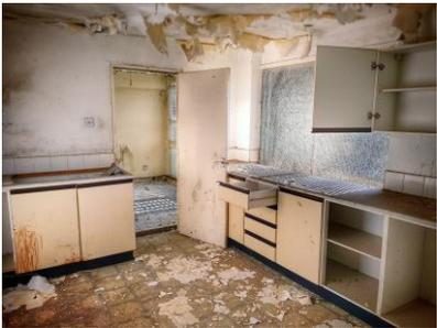
Following the asbestos removal works we then commence internal demolition which involves removing all the existing finishes and furniture, much of which is still original from the 1960's!
